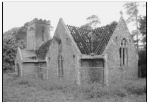
St Wandregesilius church after the fire (exterior picture courtesy of CJ Harrison)
